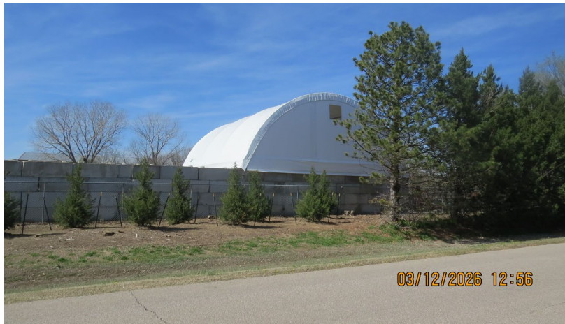
Looking west towards site and structure in easement.
