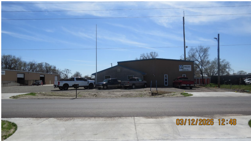
Looking south away from the site.
