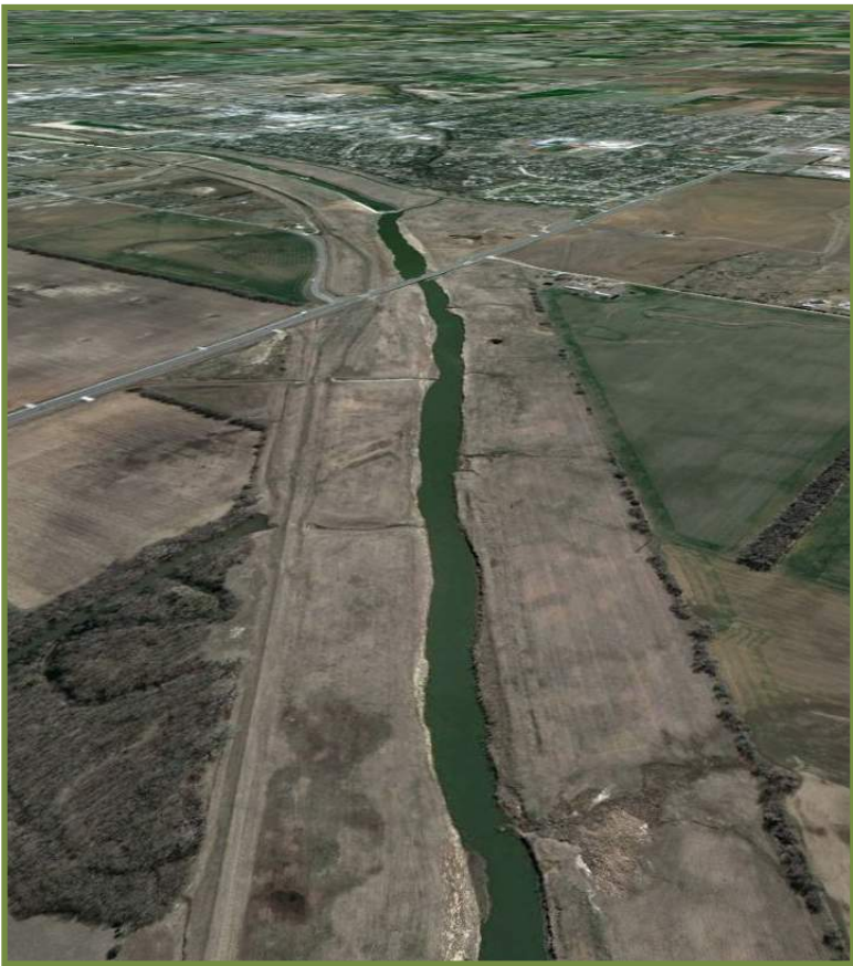
Wichita-Valley Center Floodway looking southeast
